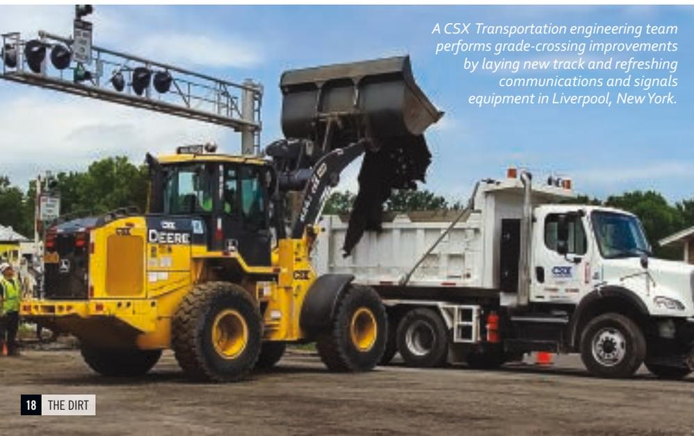
*A CSX Transportation engineering team performs grade-crossing improvements by laying new track and refreshing communications and signals equipment in Liverpool, New York.*
